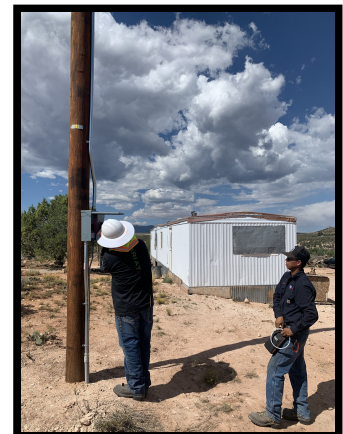
Power pole work in Westwater
