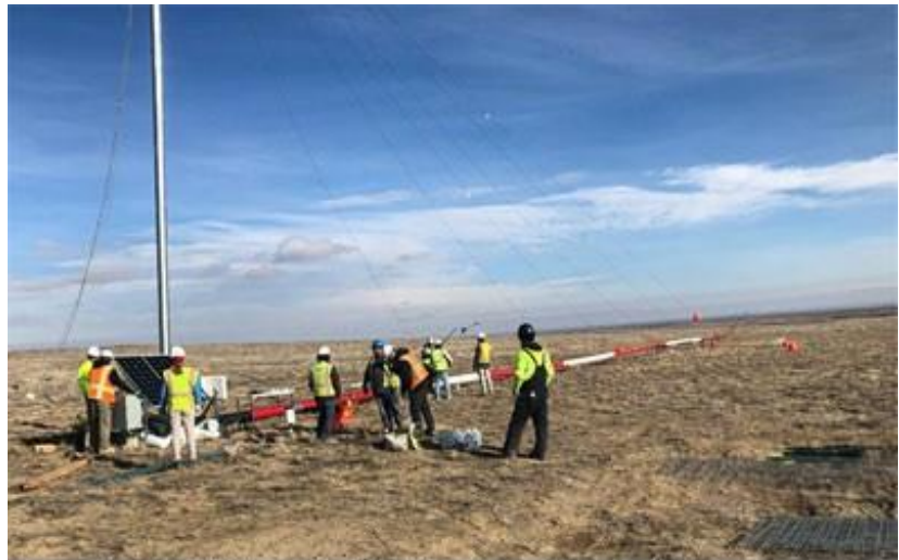
Meteorological tower under repair
